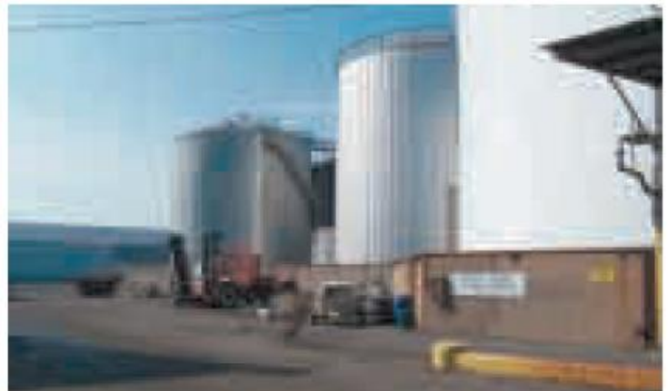
Once fully operational Innovation Fuels expects to move about 1 million gallons of biodiesel per month
